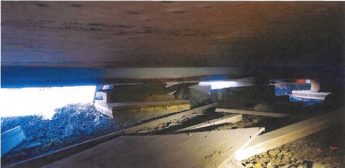
Makeshift block and wedge footings on west side
