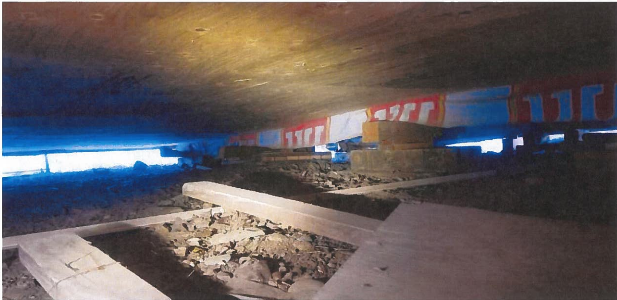
Main beam under centre of house
